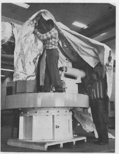
**READYING TELESCOPE** for shipment, Joe Maldonado, left, and Fred Pfeffer place specially fabricated heavy waterproof plastic bag over entire instrument. Moving parts were secured with wooden braces and steel bands. Delicate parts were packed separately.
